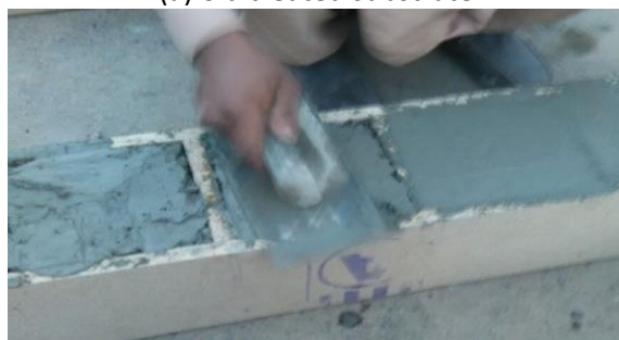
(b) Pouring of repairing concrete
